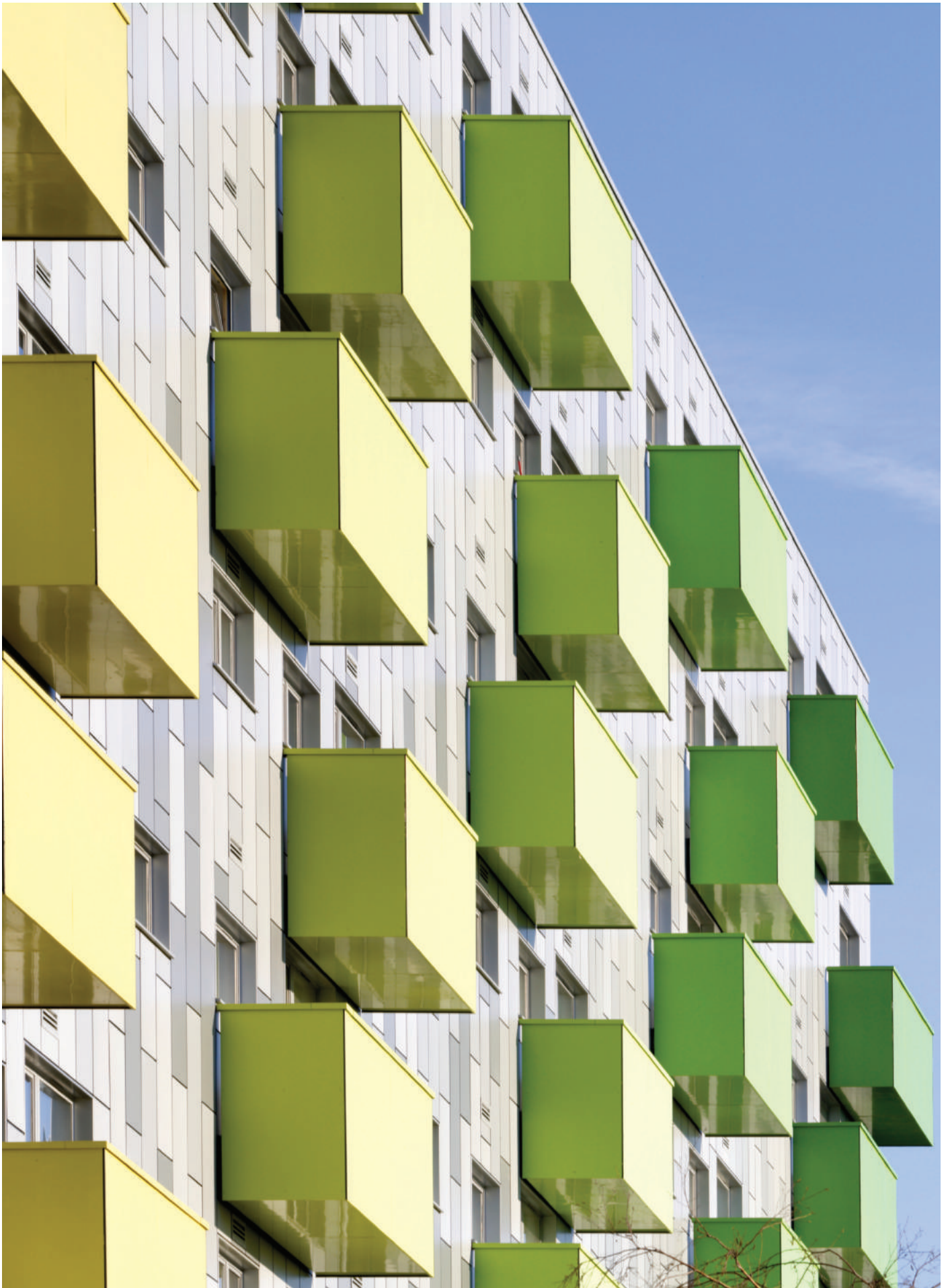
Image showing balconies of the South façade. Fading from Yellow to Green
