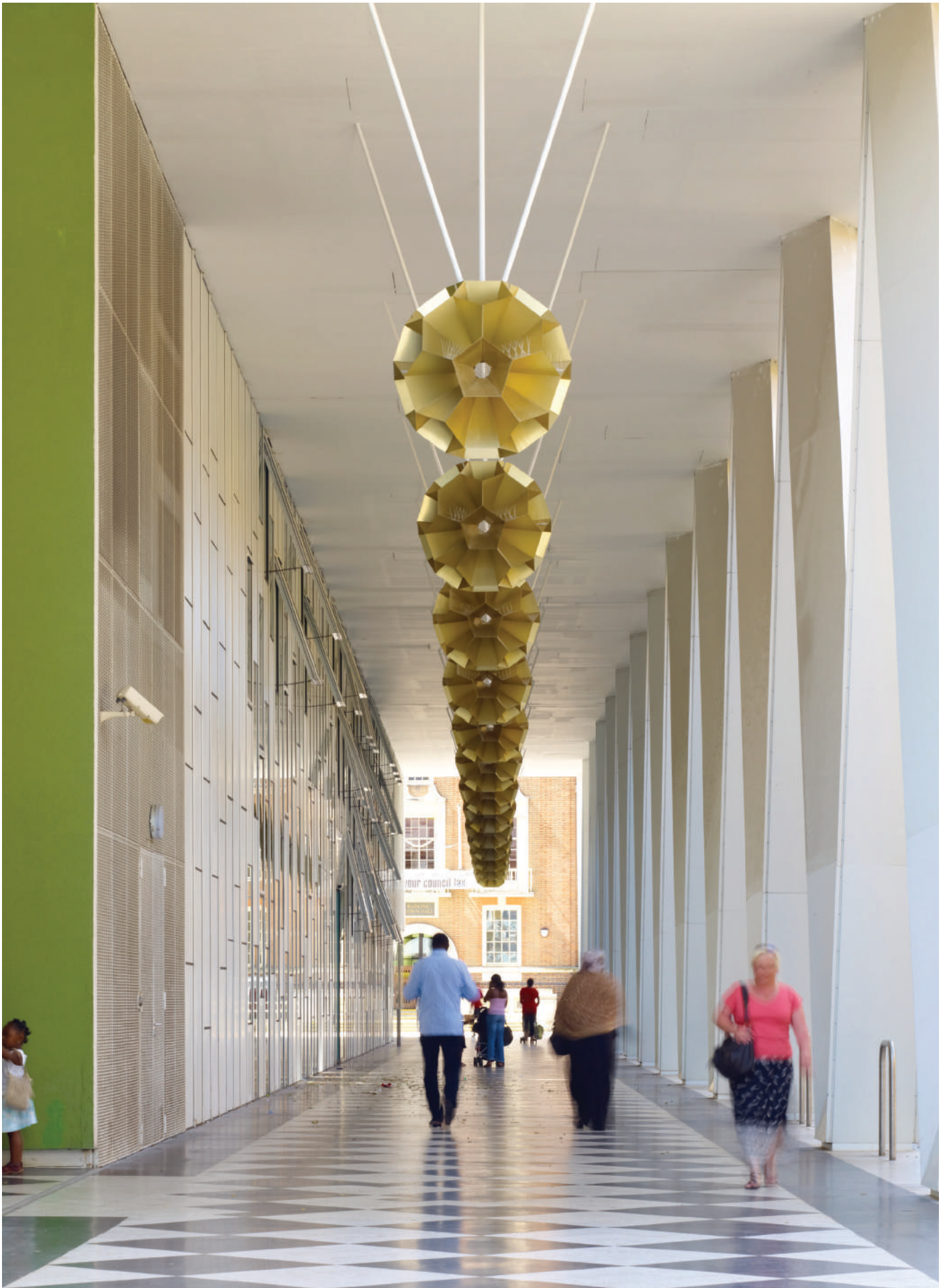
Look through Library Colonnade towards Town Hall with Tom Dixon lighting © and Colonnade designed by muf architecture/art ©
