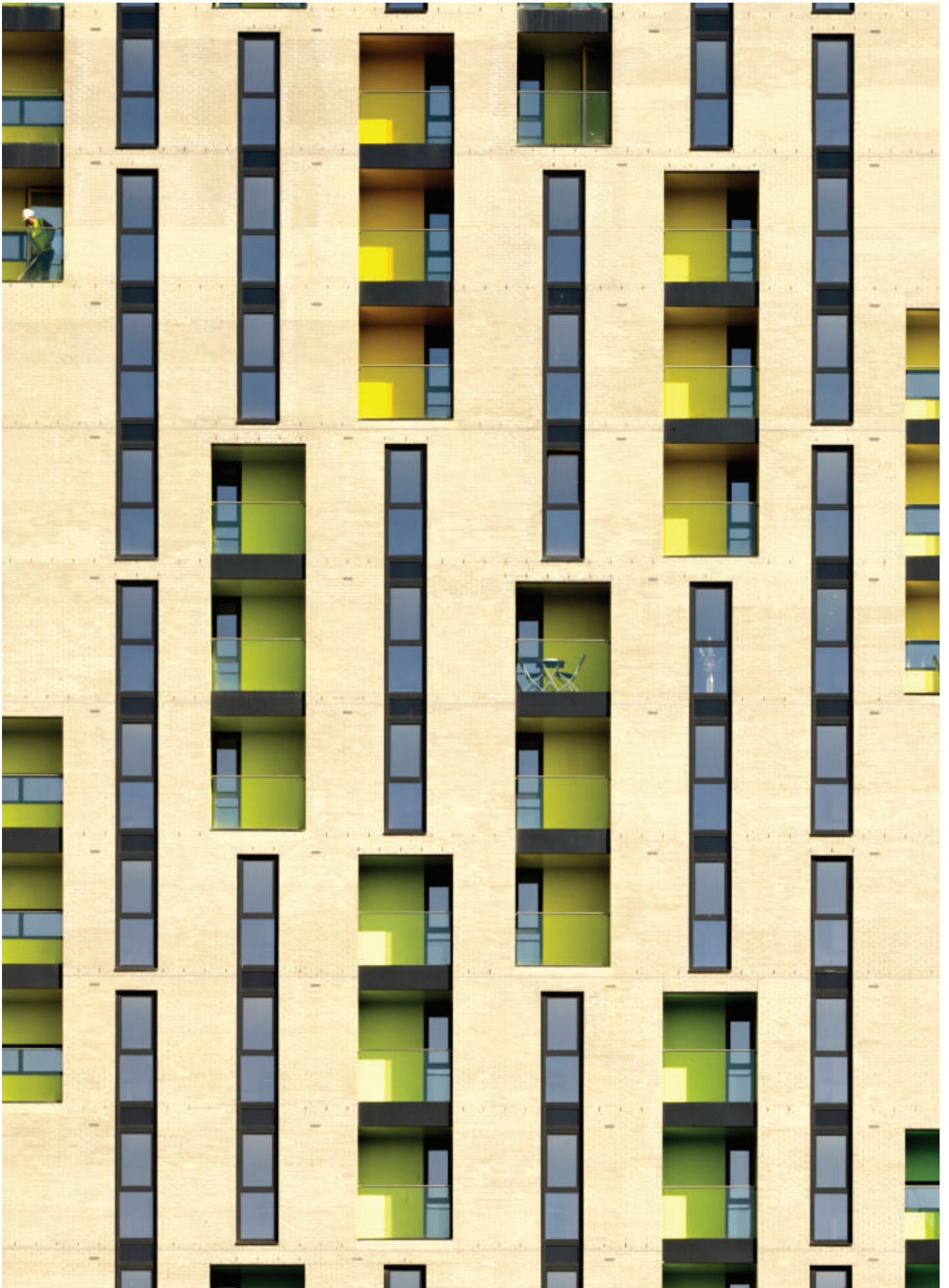
Detail view of the façade of the Lemonade Building
