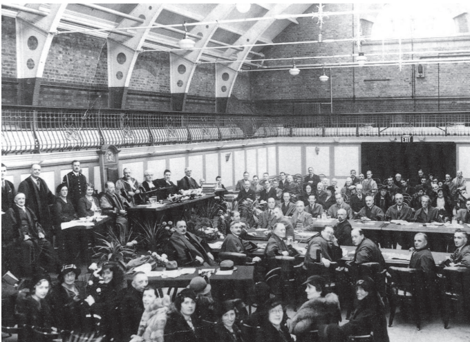
Photograph of Old Bath House, regularly used for town meetings
