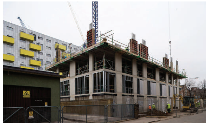
Construction of Bath House
