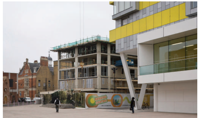
Construction of Bath House
