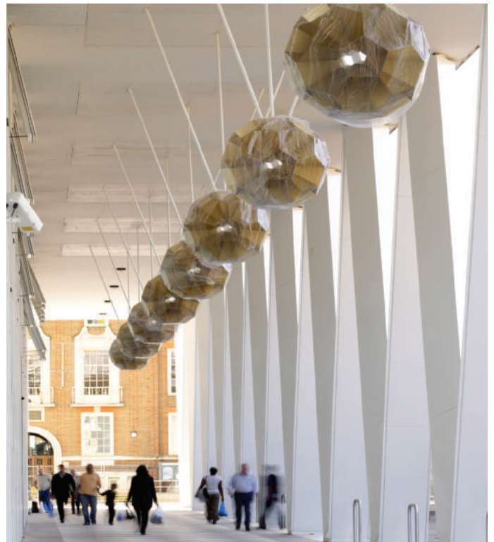
Barking Central colonnade with Tom Dixon lighting
