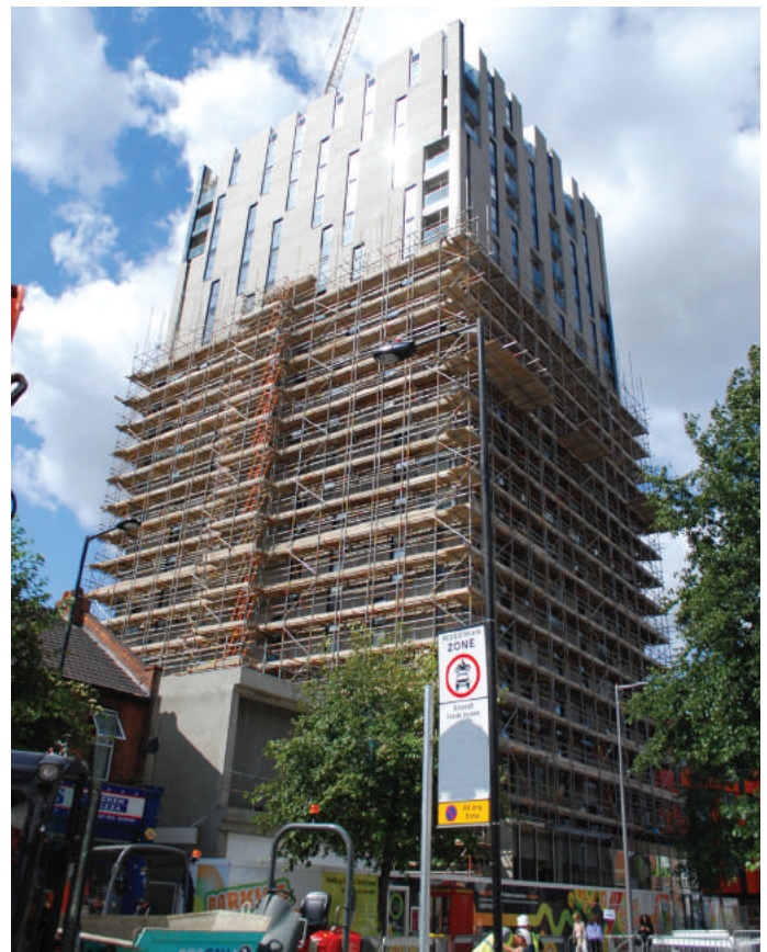
Construction of Lemonade Building cladding
