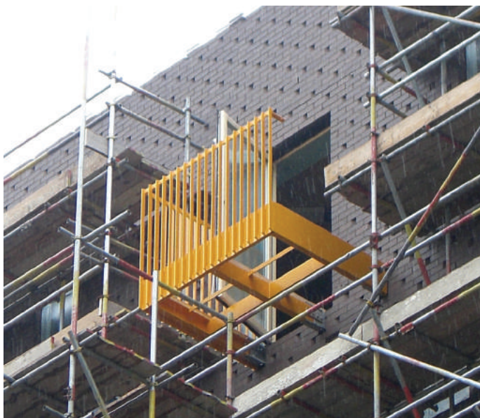
Construction of Bath House balconies
