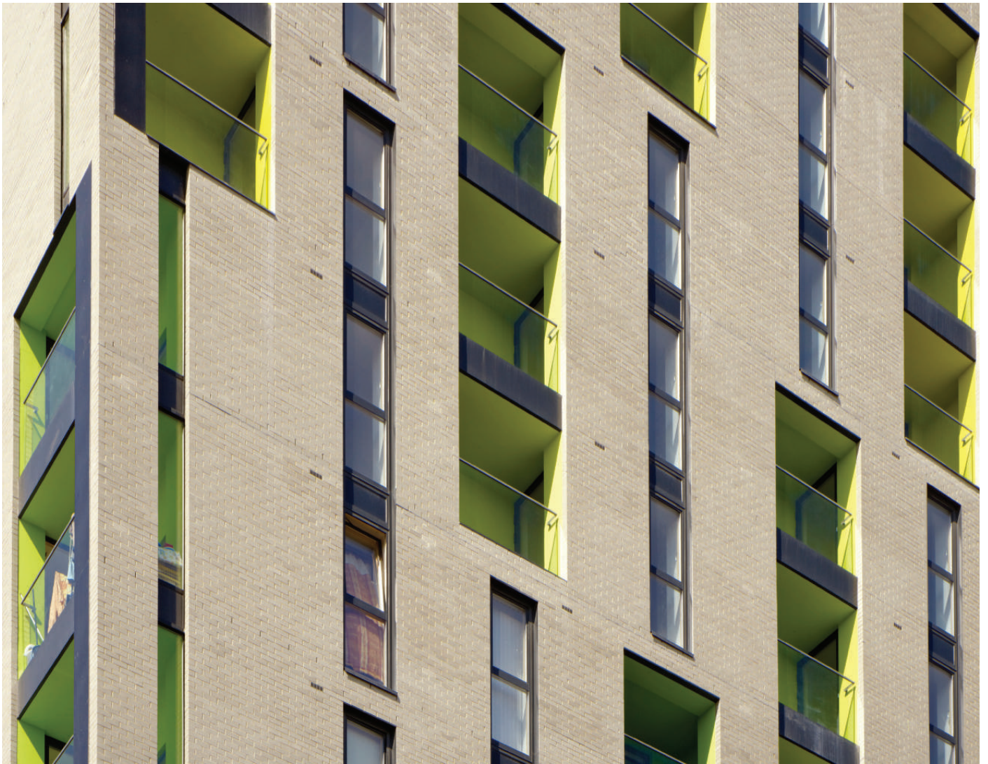
Detail view of the façade of the Lemonade Building
